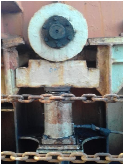
Gambar 3. Kebocoran Jack Hydraulic
