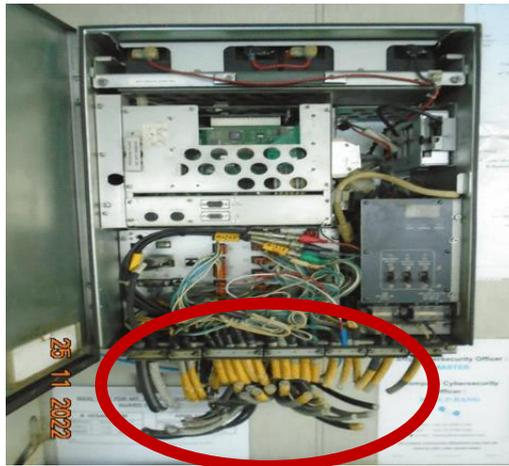
Gambar 5. Kerusakan *Bridge Navigational Watch Alarm System* (BNWAS)
