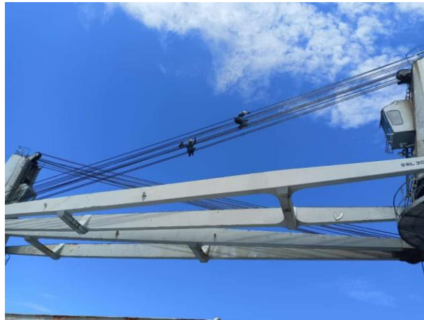
Gambar 6. Regreasing Wire Crane
